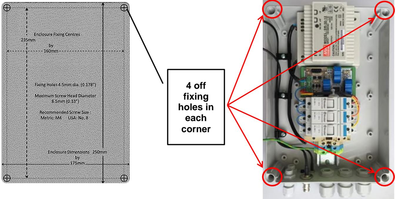
If the fixing screws are not in a convenient position for the surface on which the controller is to be fixed then the use of rails, frames or battens is recommended.
